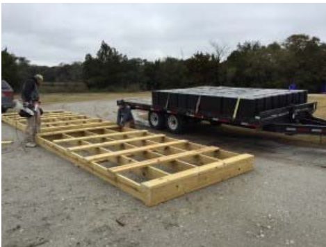
New Floating Dock Construction, February 2015
